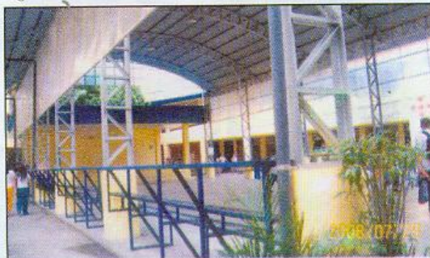
The Php 4.3-million new covered court at Dr. Josefa Jara Martinez High School is a modern structure that can accommodate a big crowd during graduation and other important school events. This is a project of then QC Councillor Neneng Montilla through the request of Dr. Victoria B. Mangosong, school principal.
