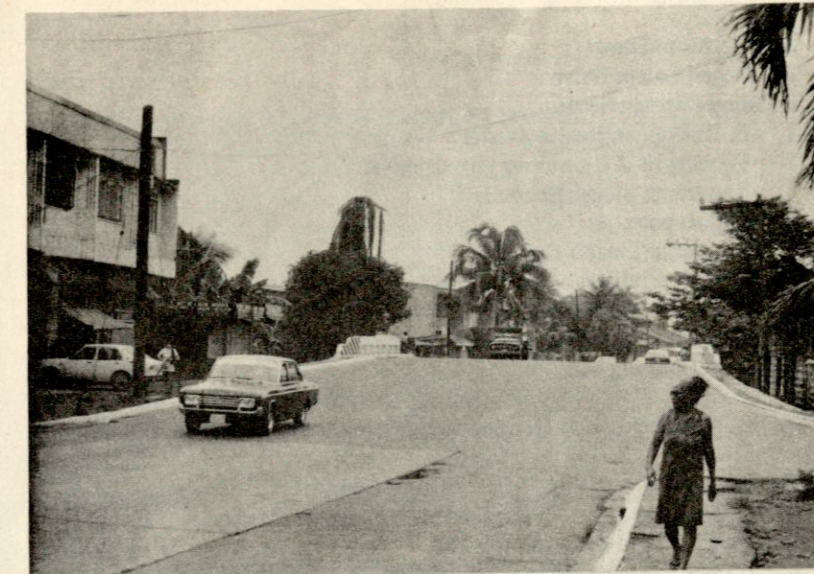
The Newly Completed Victoria Bridge
