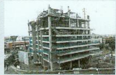
Tower 1 should be completed by mid 2006
