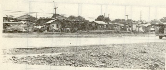
The structures to be demolished at the road right-of-way of the Don Mariano Marcos Avenue.
