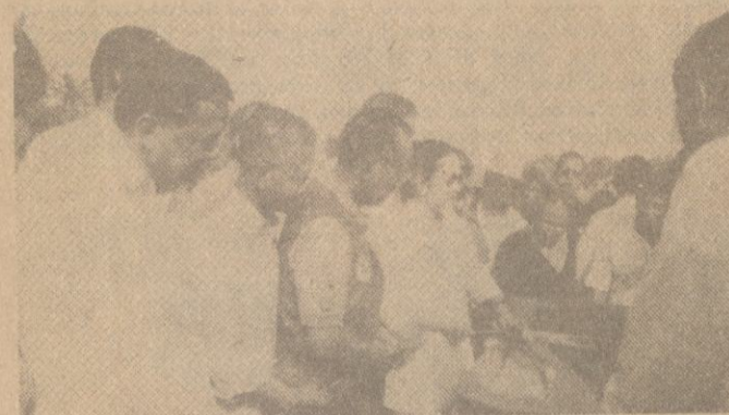
In December last year, President Ramos led government officials in unveiling the marker of the newly completed Katipunan Road Extension and the Flyover at the Aurora Blvd. Intersection which were expected to decongest traffic near Ateneo. With the President were Mayor Mathay, Public Works and Highways Secretary Gregorio Vigilar and Senator Anna Dominique Coseteng.
