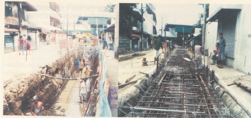
SOME OF THE CITY-FINANCED, COMPLETED DRAINAGE IMPROVEMENT AND FLOOD CONTROL PROJECTS 2003-2004
